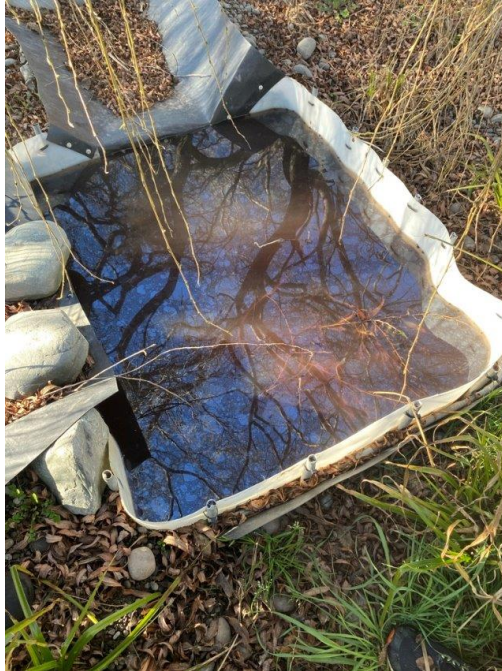
Figure 5. Picture of the third pond outlet, lack of surface flow has allowed the water in the bucket to become stagnant.
