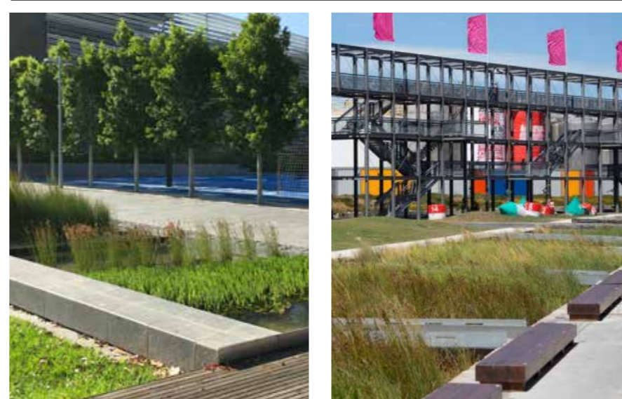
Stormwater: making surface water collection visible
